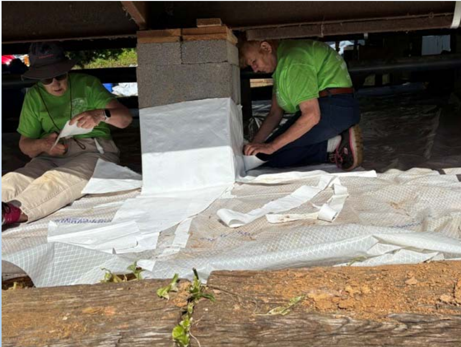
Betsy and Margie worked on wrapping the support pillars with additional moisture barrier.
