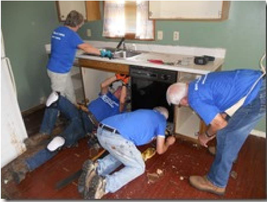
Bobbi Trick, Chuck Shelton, Brian Schroeder, and Russ Rankin remove rotted kitchen sink
